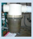
Wet vacuum system: Change pump screen as needed or directed by manufacturer. Seal plastic container with screen and contents (including any water that may be present) and store with amalgam waste. Do not rinse contents down sink or other drain.
