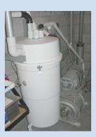
Dry vacuum system: Have a qualified maintenance technician, amalgam recycler, or hazardous waste disposal service pump out and clean the air-water separator tank.
