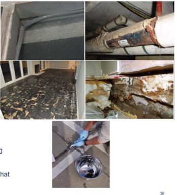
The materials were prioritized by developing six factors that relate to the load or mass of PCBs associated with the materials, the likelihood of the material to get into stormwater during the demolition process, and the relative difficulty to remove the material from the building. A spreadsheet was used to assign a score to each material based on the factors, which were evenly weighted. The materials were then ranked and the highest scoring materials selected.
